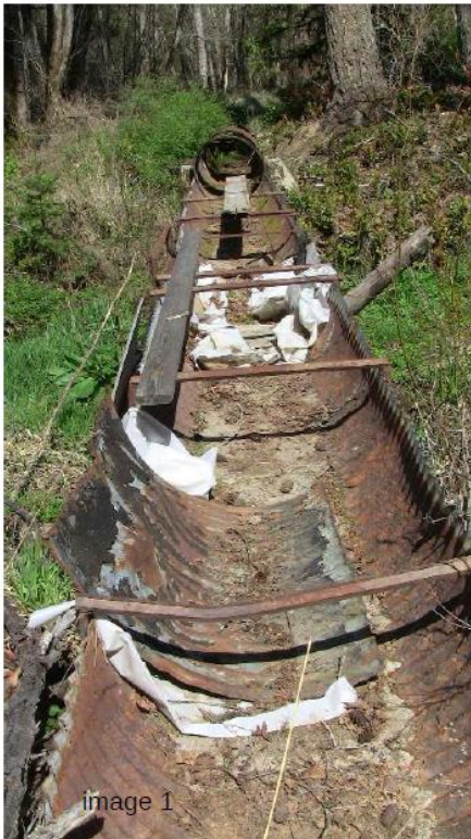
Figure 7. Main flume for fish release if they are entrapped in the ditch. Plastic sheet indicates release hole opening.
